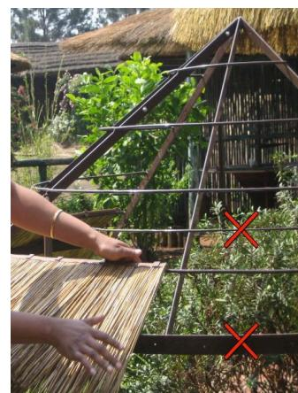
**Step 5:** Place the roof cone along the outer centre ridge of the frame, if necessary with the aid of a broomstick. For large diameters, you can first place the roof cone on the frame and raise it to affix the last reed panels. To keep the cone in place, attach it to the frame with the ties provided for this purpose.
