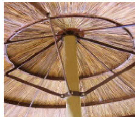
**Step 5:** Place the roof cone along the outer centre ridge of the frame, if necessary with the aid of a broomstick.
