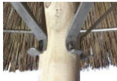
**Step 4:** Clamp the reed panels with the hooks fitted along them to the outside of the metal rings: begin with the second row from the underside of the incline. The lowest ring serves as a support for the reed to rest on. Tip: lay the thickest reed or makuti panels to one side for the highest row.
